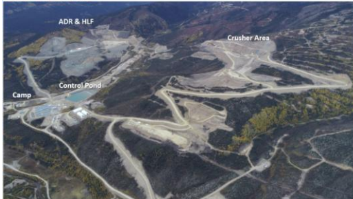
Overview of Site
